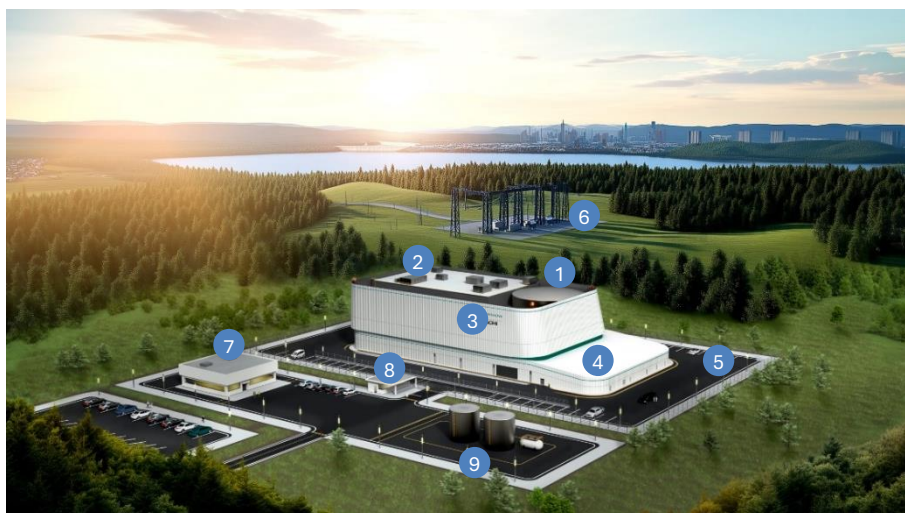
1 – Reactor Building; 2 – Turbine Building; 3 – Radwaste Building; 4 – Control Building; 5 – Protected Area; 6 – Switchyard; 7 – Admin Building; 8 – Security Building; 9 – Tanks & Skids
